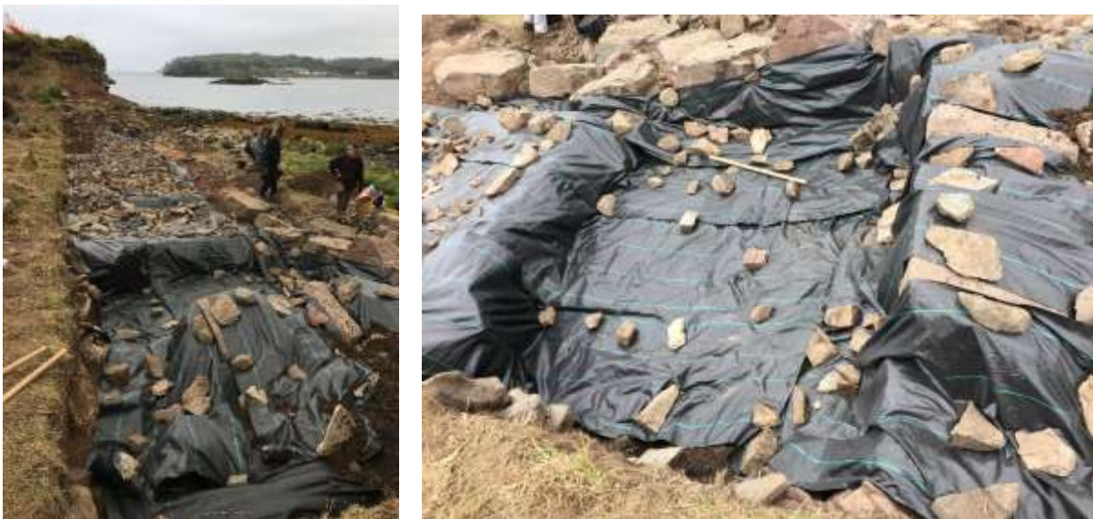
Figure 34 Laying of geotextile across excavated trench
