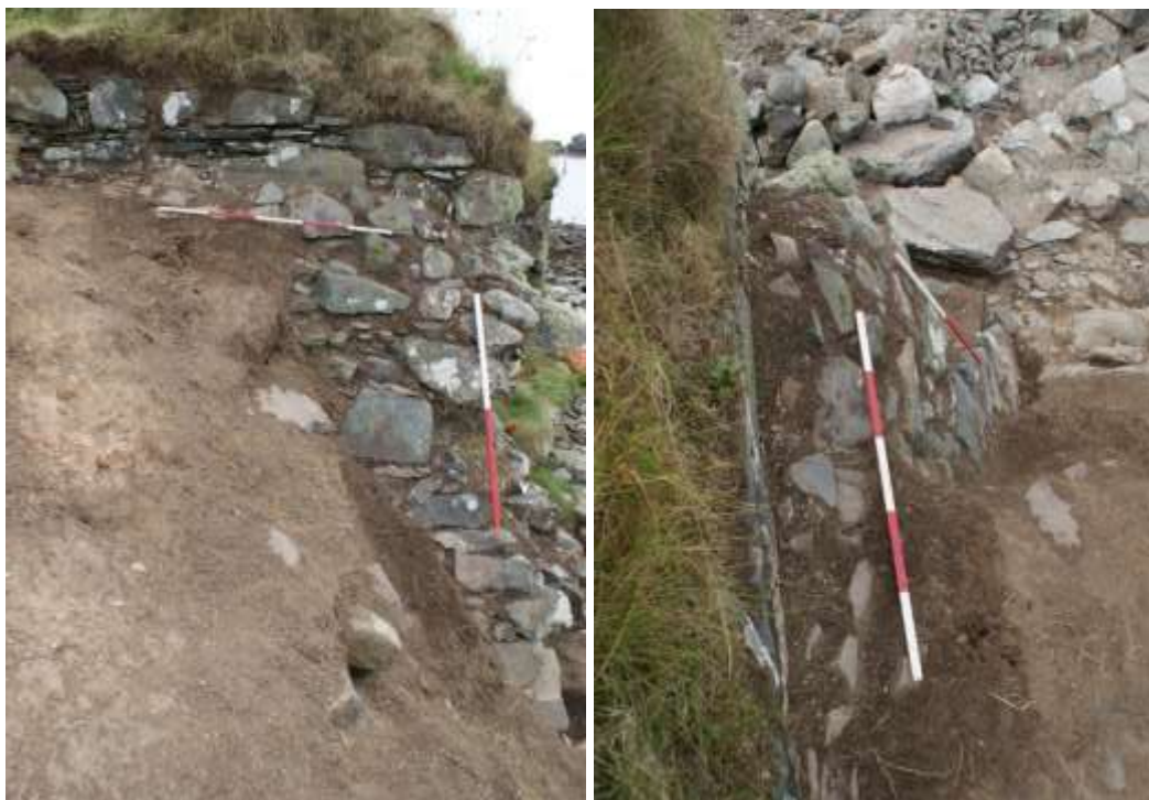
Figure 12 Exposed part of batter or buttress (7017) from the north (left) and from above looking west and showing how it abuts face of curtain wall (7029) at the top.
