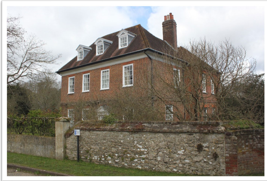
(Fig 15: Court Lodge; outbuildings to the east provide information about the churchyard wall and its phasing)
