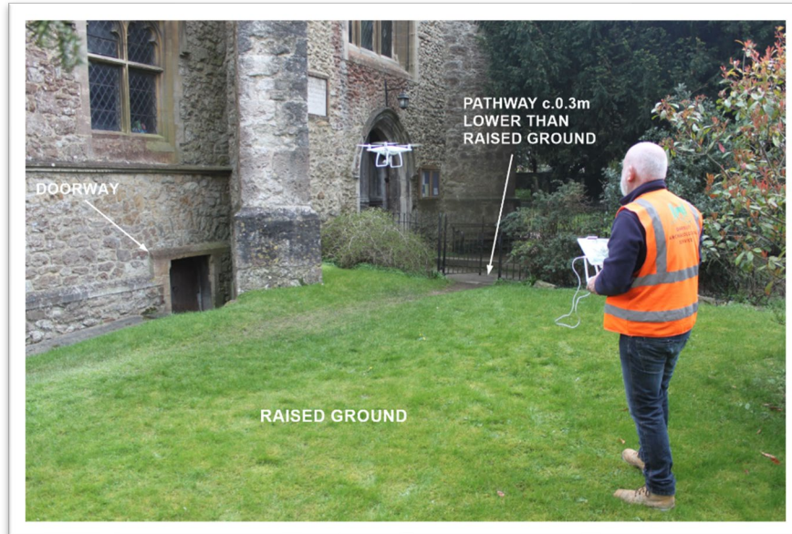
(Fig 31: Looking south-east from PDS across raised churchyard at West Tower and frontage)
