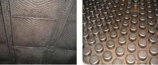
In order to avoid droplets in off gas there is a mesh grid on absorber top Absorber contains 10 trays
