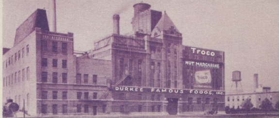
Chicago Refinery at Elston Ave. and Logan Blvd.
