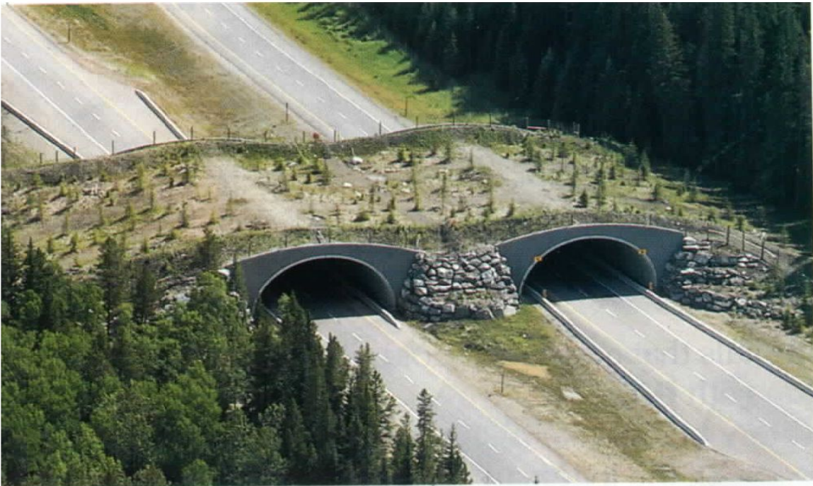
One part of the Trans-Canada Highway that runs through Banff National Park in Alberta, Canada was once called "The Meatmaker" because so many wild animals were killed there. This wildlife bridge was built there as a solution to that problem.
