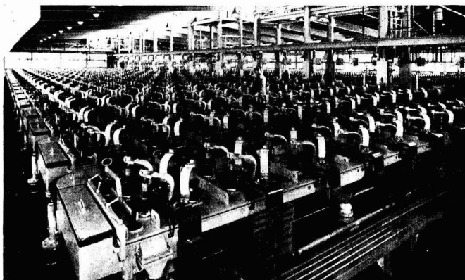
New mercury cell installations of Murgatroyd's
