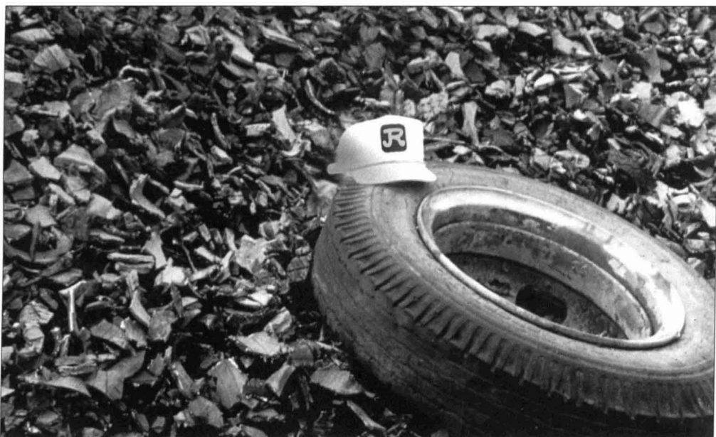
Chipped tires comprised the underlying drainage layer of the cap.
