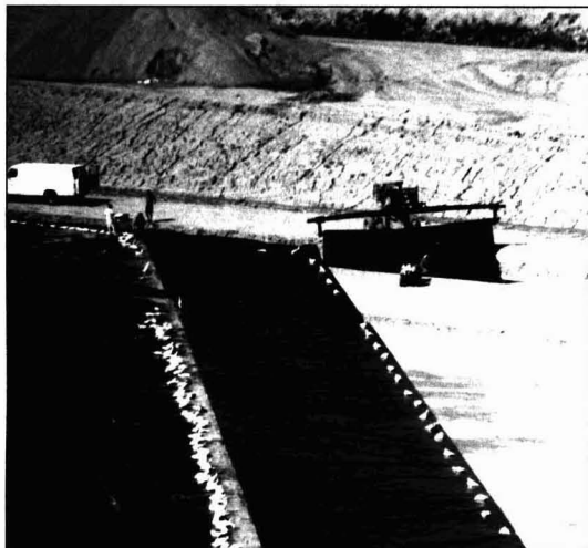
Above: The new 60 mil HDPE liner is put down and then covered with soil. Right: Ground is prepared for the new landfill.
