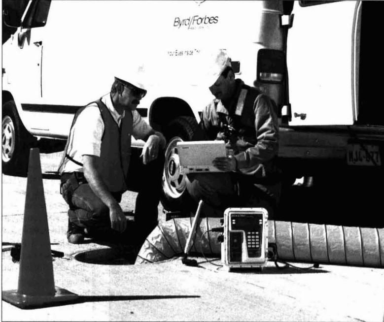
Flow meters were installed to "get the heartbeat" of the collection system.
