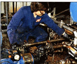
Metering Pumps and In-Line Mixers
