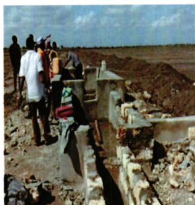
Boji farmers' irrigation project division chambers rehabilitation & furrows development ongoing
