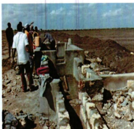
Boji farmers' irrigation project division chambers rehabilitation & furrows development ongoing
