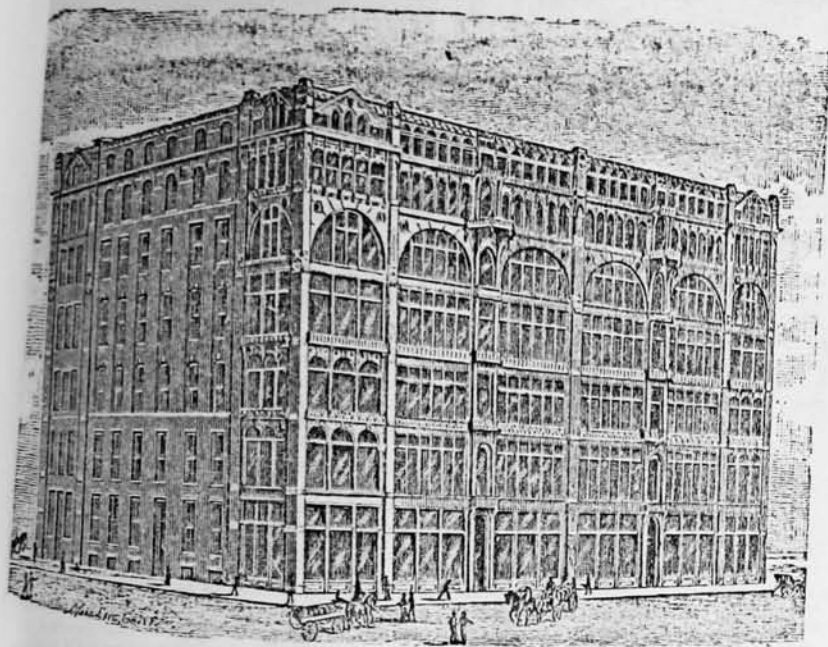
WARNER'S SAFE REMEDIES BUILDING.
