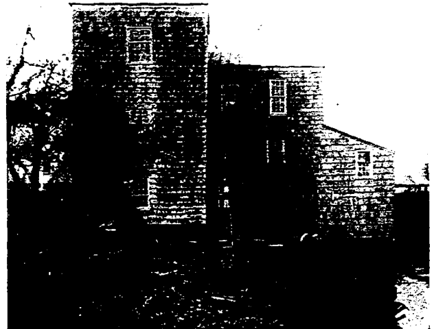
Watermill, Water Mill, L. I., original one built by Edward Howell in 1644-5
