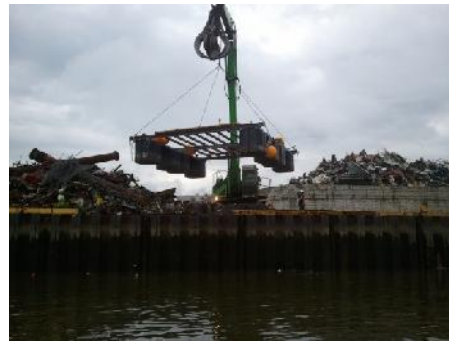
Figure 3. Lowering the assembled raft into the water.
