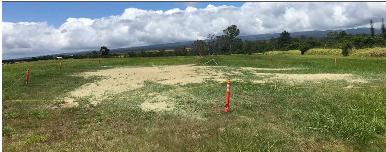
Figure 12. Sediment disposal site, marked by cones, after hydromulch application.
