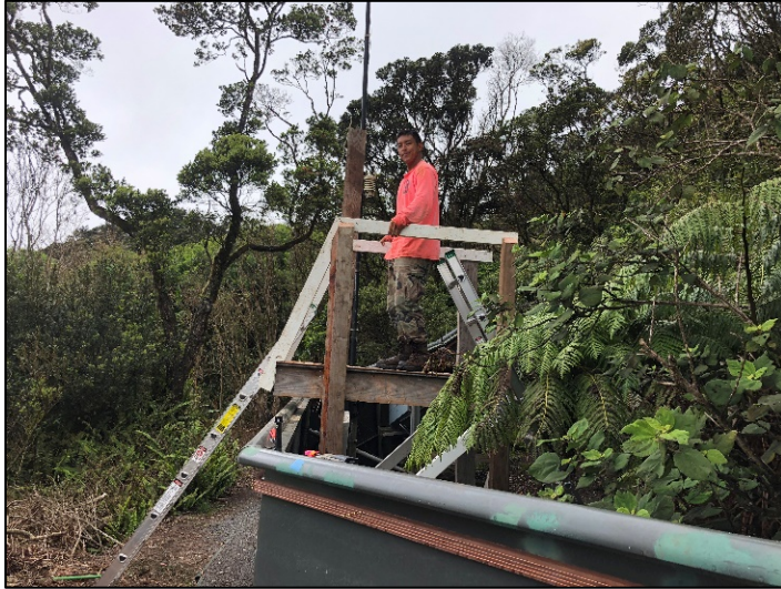
Figure 27. Built-in crossover at Palikea South enclosure reduces the risk of E. rosea getting into the enclosure from the ladder.
