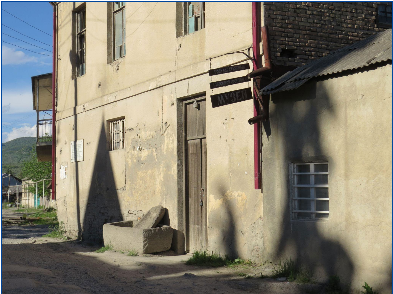
Figure A1.71: Old building of the Museum of Local History in 2014 © Didi Liakhvi Valley Museum-Reserve
