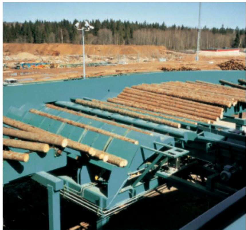
Stora Enso continues to invest in its sawmilling operations in Russia. Annual capacity at Nebolchi Sawmill will be doubled to 220 000 m 3 .
