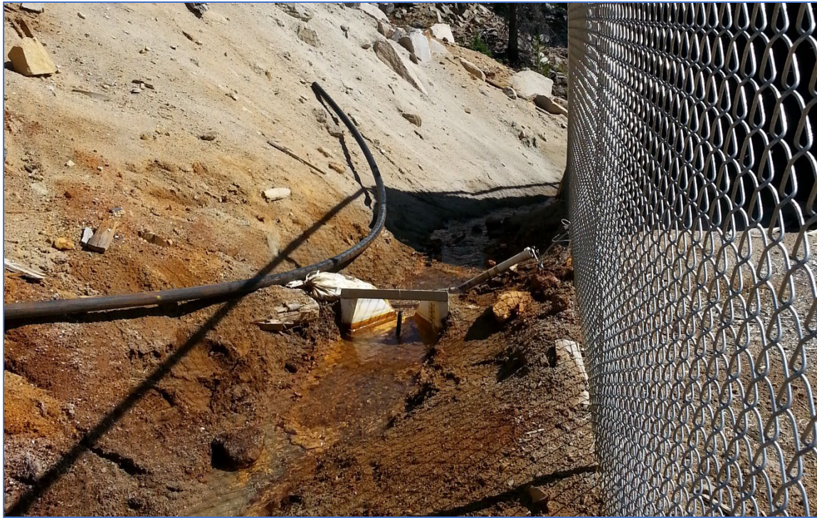
Figure 3. Crystal Mine flume located approximately 20 yards downgradient of the adit.
