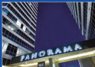
Panorama Towers 137 MOBOTIX Kameras, USA
