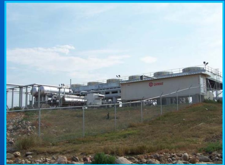
22 MW OREG 1 Power Plant North Dakota
