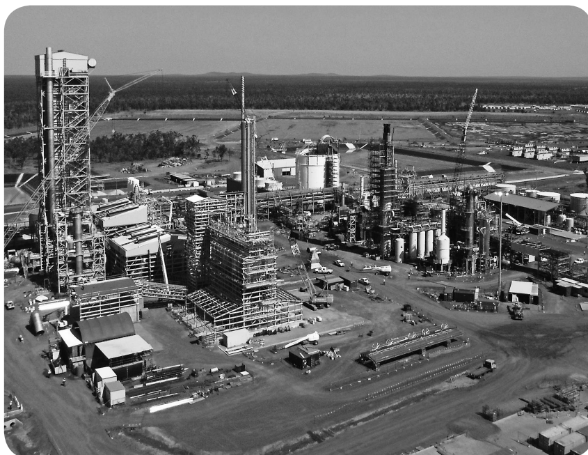
Moranbah ammonium nitrate manufacturing complex currently under construction (October 2011).
