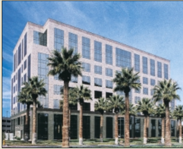
Commercial development activity continued in Las Vegas with the opening of 3993 Howard Hughes Parkway, a new eight-story, class-A office building.
