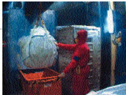
Asbestos removal at the Berlaymont building - Brussels.
