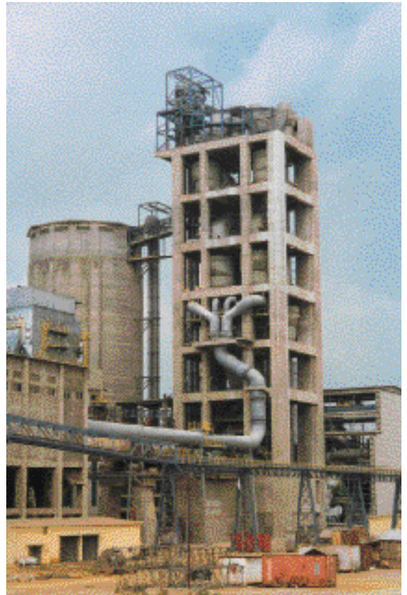
But Son cement plant - Vietnam.
