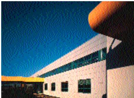
Amboise pharmaceutical production unit France.
