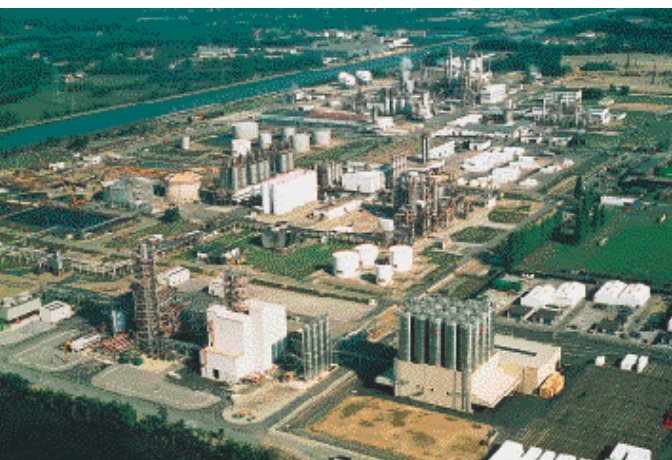
Geel PTA plant - Belgium.
