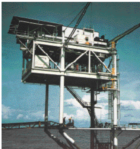
MOSS platform - Gulf of Mexico.
