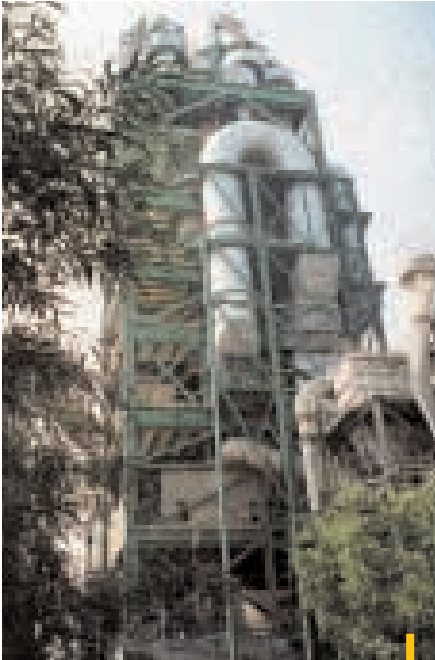
Cement plant at Bouskoura (Morocco).
