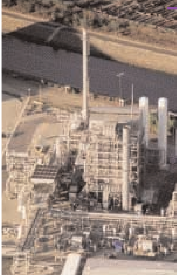
Hydrogen unit at Carson, California (U.S.A.).
