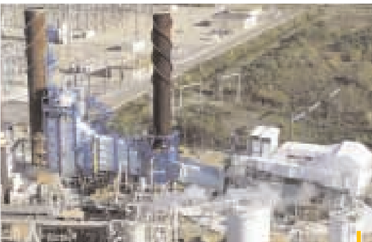
Cogeneration unit at Fos-sur-Mer (France).
