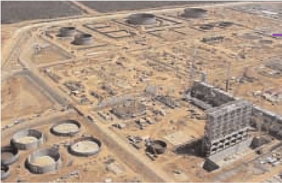
Overall view of the SINCOR jobsite at Jose (Venezuela).
