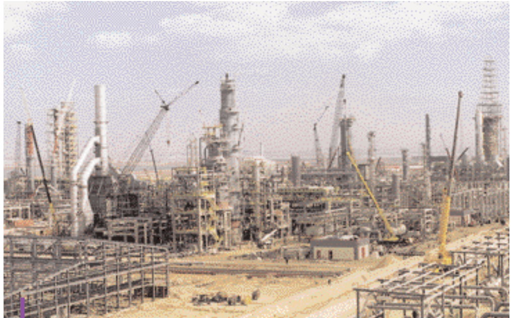
Overall view of the MIDOR/MIDTAP refinery (Egypt).
