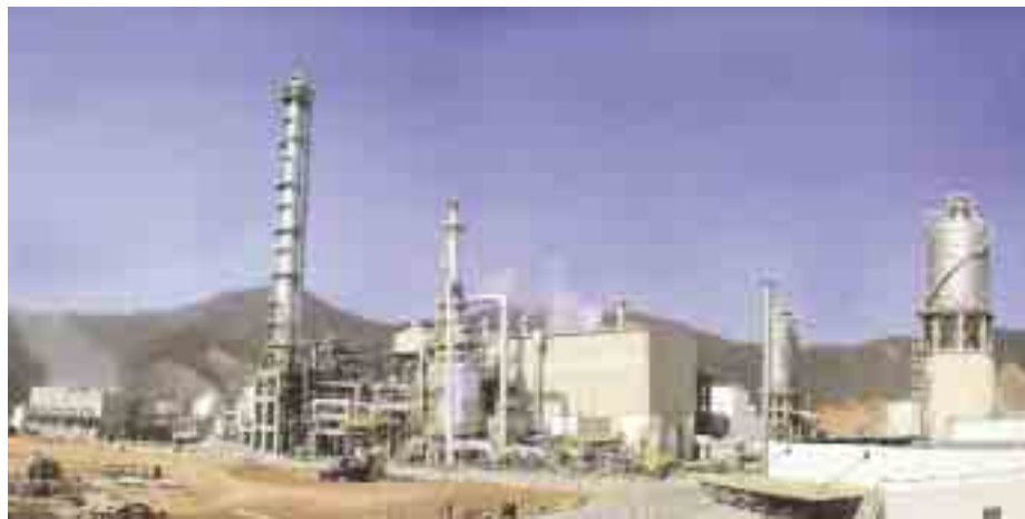
The PTA plant in Zhuhai, China.
