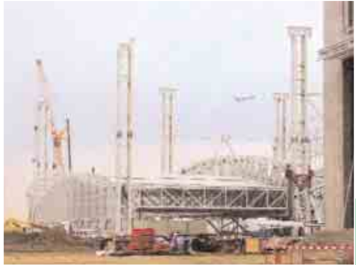
The Airbus A380 assembly plant under construction in Toulouse, France.
