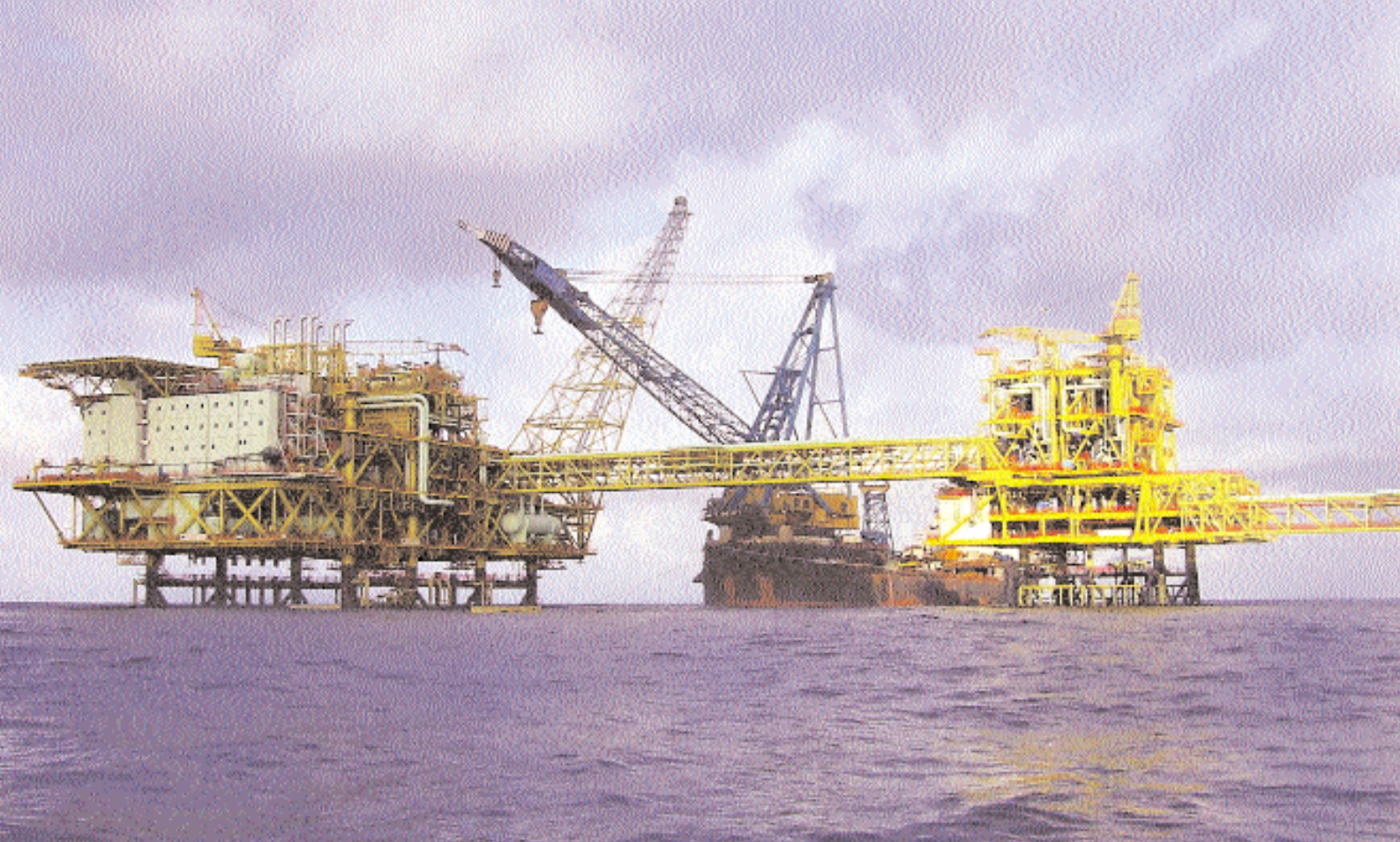
The central platforms of Cakerawala field, Malaysia / Thailand.
