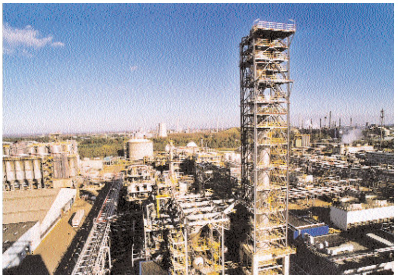
The polypropylene plant "PPF6" at Geleen, The Netherlands.
