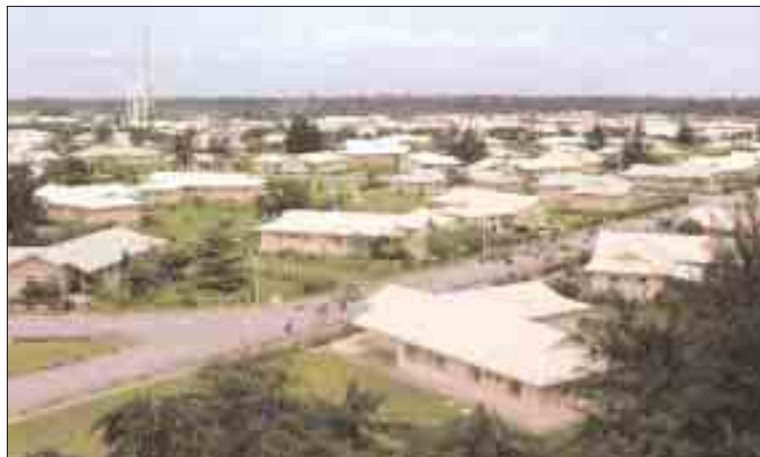
The residential area designed and built by Technip-Coflexip at Bonny, Nigeria.
