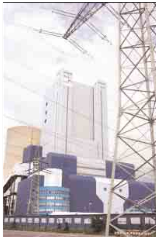
The power plant of Niederhausen, Germany.
