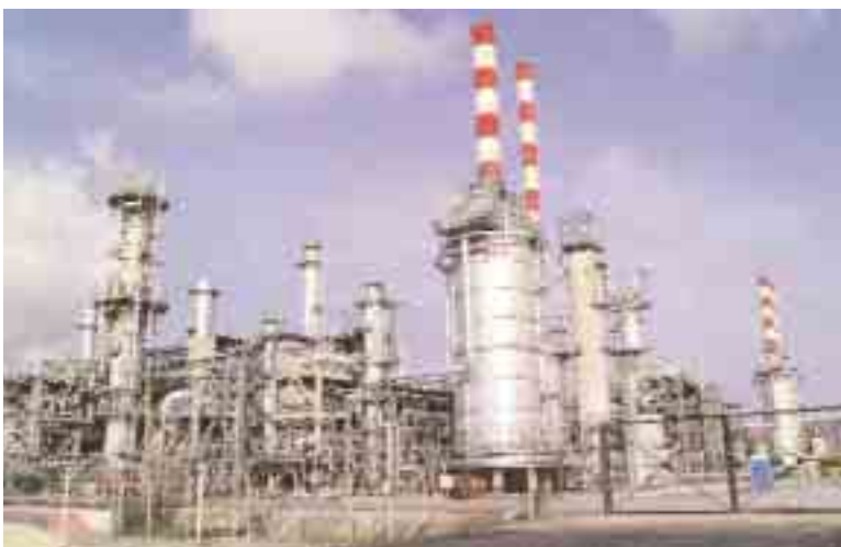
One of the LNG trains at Bonny, Nigeria.
