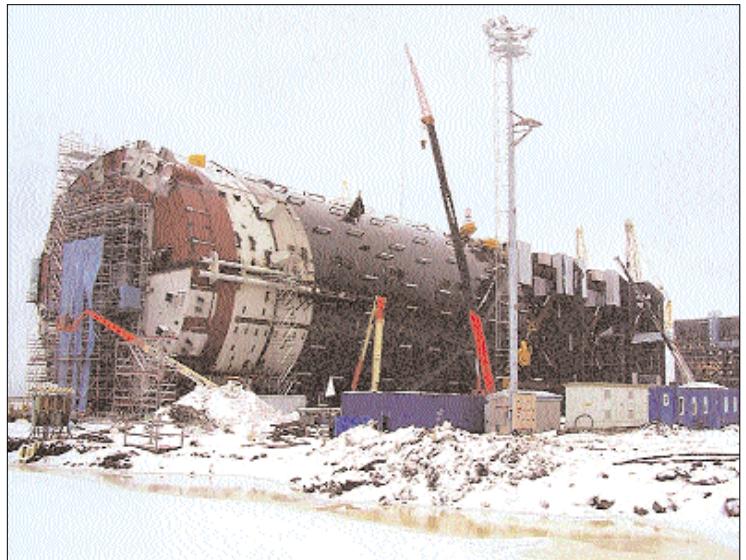
The Gunnison Spar's hull under construction in Mantyluoto.
