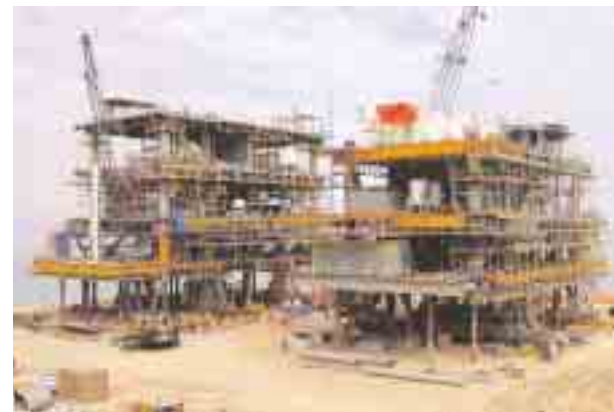
Soroosh & Nowrooz platforms under construction.
