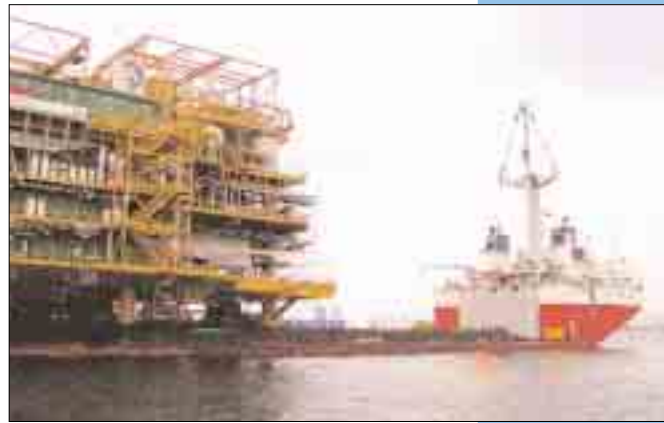
Load out of the Amenam platform, Nigeria.
