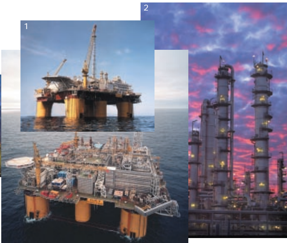
2. Phenolchemie designed this phenol and acetone manufacturing facility near Theodore, Alabama USA using Plant Design System (PDS™), INtools™, and SmartPlant® Review. (Photos by Bernd Billmeyer)
