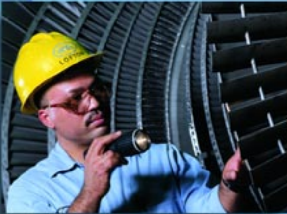
During 2004, a new dense pack turbine was installed on Stuart Station's Unit 4. The dense pack rotor has an aerodynamic design that essentially grabs more steam, improving the heat rate and fuel efficiency of the unit. Here, Lawrence Lofton, Equipment Mechanic, inspects a turbine rotor.
