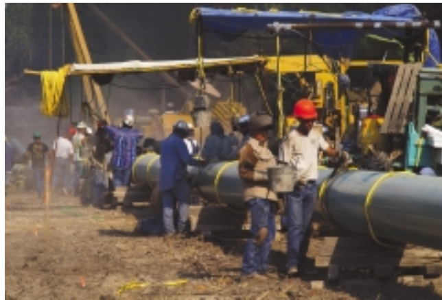
Pipe gang welding in Cameroon
