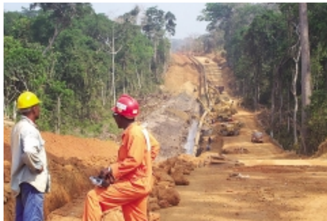
Lowering-in pipe in Cameroon
