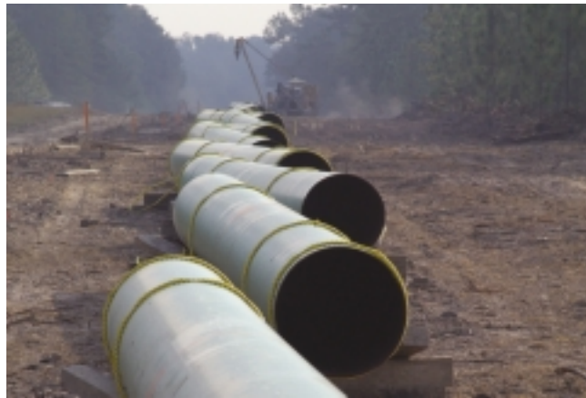
Pipe strung along the Right of Way in Cameroon
