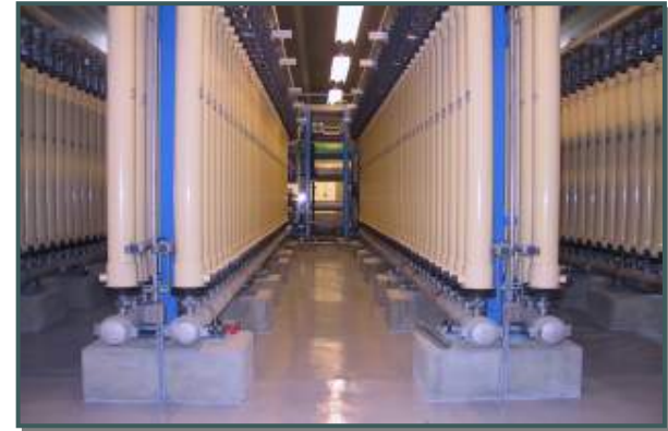
Pall Aria™ membrane systems remove pathogens from source water to meet drinking water regulations
