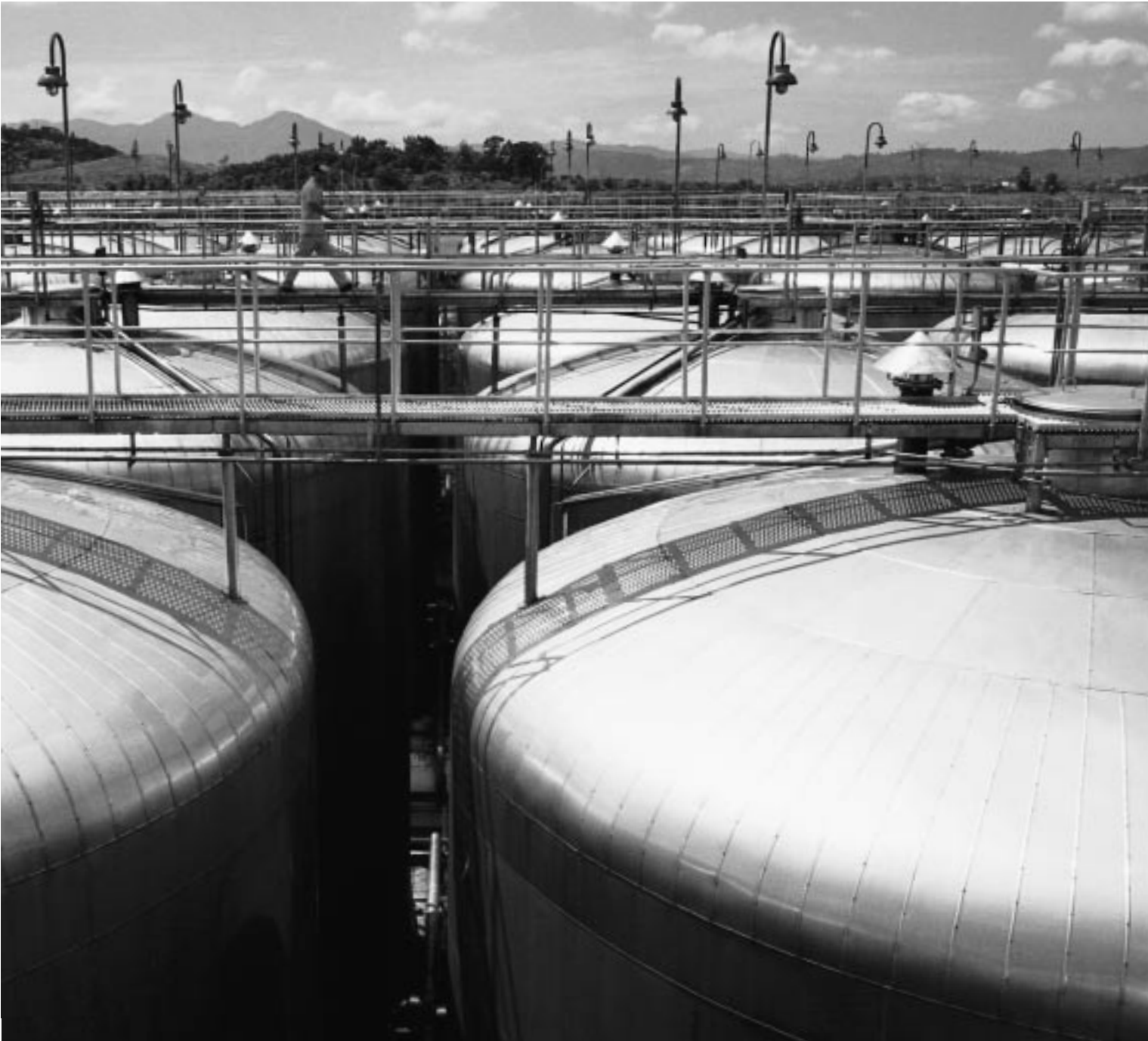
AmBev's highly efficient Nova Rio plant in the state of Rio de Janeiro represents 20% of the company's production.
