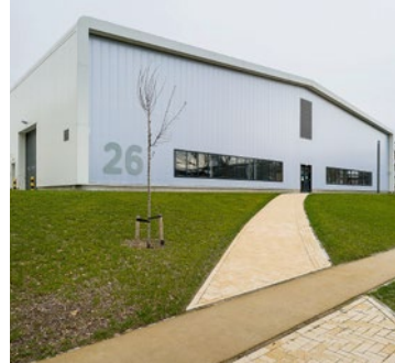
The new distillation plant in Geleen, Netherlands now is open.
