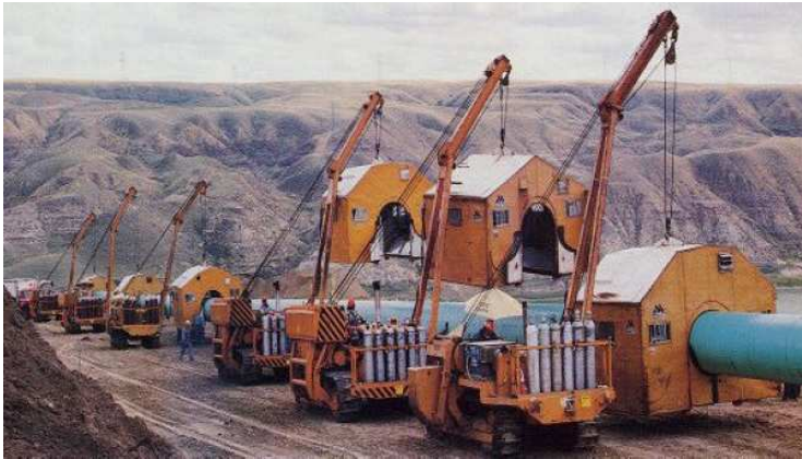
Figure 2-1: Main Line Joints
