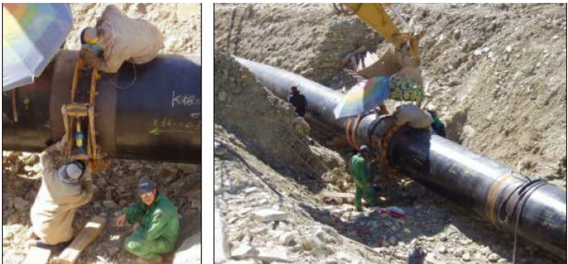
Figure 2-2: Typical Tie-In Welding Arrangement for new construction
