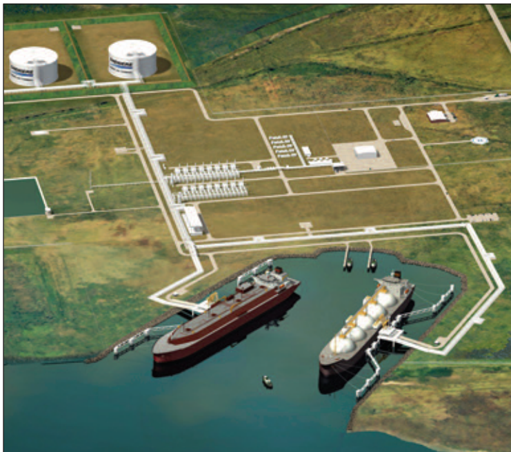
An artist's impression of the Sabine Pass LNG terminal to be built in Louisiana, USA.
