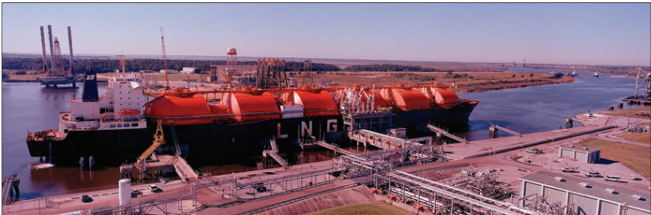
The USA is seeing a surge in LNG imports. Lake Charles, Louisiana is one of the country's existing reception terminals, all of which are being expanded to help meet fast-growing LNG demand.
