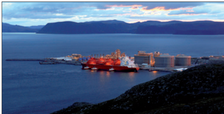
Gas from the Snøhvit field is piped to a liquefaction plant at Melkøya for export as LNG.
