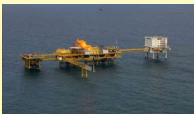
◀ Gas flared on a platform in the Rio del Rey basin
