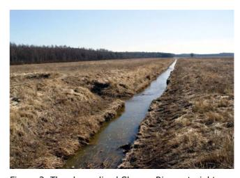
Figure 2. The channelized Slampe River, straightened in the 1970's draining the floodplain with abandoned grassland, photo taken in 2004 before the restoration activities. Photo: G. Pāvils
