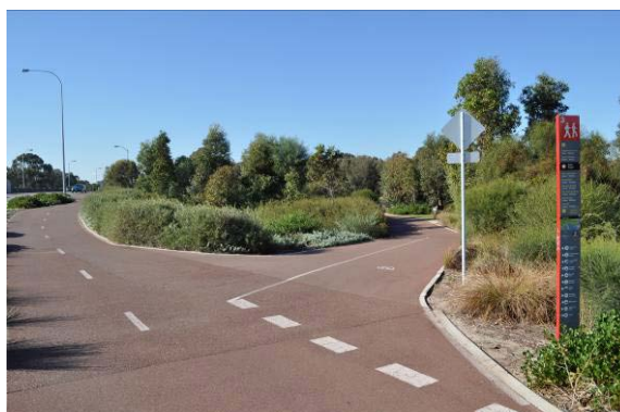
SMC2 – East Entrance: Overpass entry
