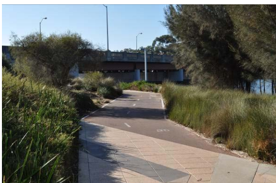
SMC2 – East Entrance: Bridge underpass entry
