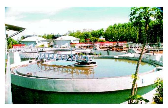
Fig-47. A view of Sewage Treatment Plant (Primary Clarifier) in Hardwar
