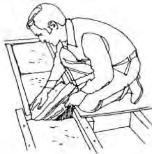
Install ceiling insulation
