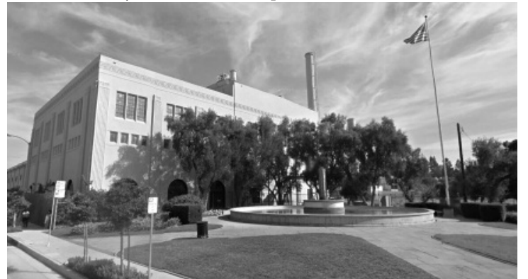
Pasadena's Water and Power Department
