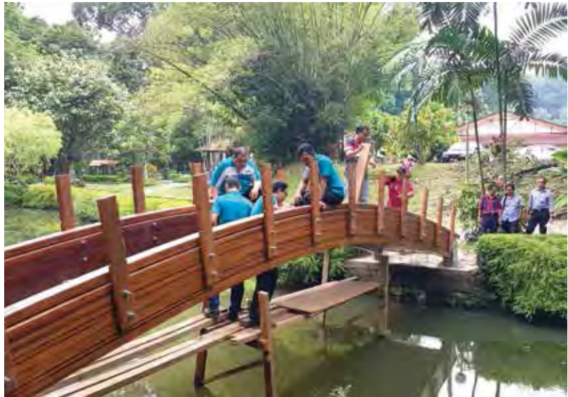
Pemasangan komponen jambatan Assembling of bridge components
