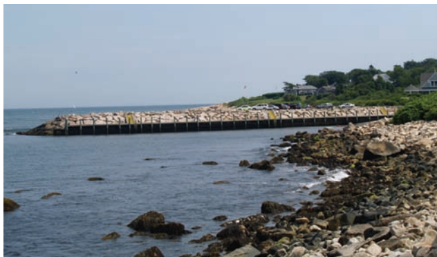
Figure 8.16. This bulkhead at State Pier #5 in Narragansett provides a sheltered cove to tie up, launch a boat, fish, or scuba dive. Human-made structures are designed to prevent erosion and provide sheltered areas for human use. Photo by Malia Schwartz.
