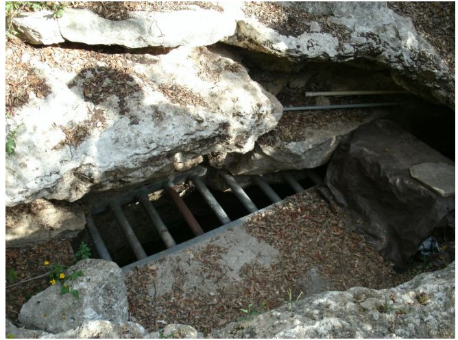
Figure 3. Concrete gate at Ezcell's Cave Credit: Jim Kennedy
