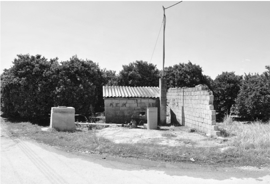
Figure 2.3 Borehole irrigation pump located just west of Neo Ireo (Chronika), 2012. Photo: C. Witmore.
