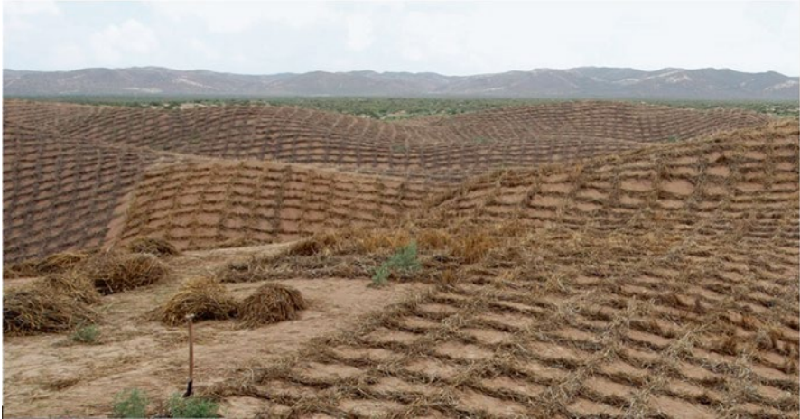
Fig. 4.9 Making straw checkerboard on dunes to stabilize them (Photo courtesy of Michael Reynolds)
