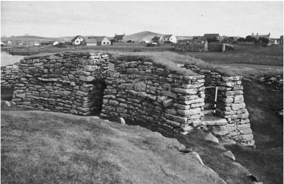
FIGURE 5.25 Clickhimin, Shetland, view of blockhouse, A (above), from the enclosing fort wall, B (below), from within, showing scarcement
