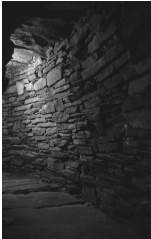
FIGURE 5.2 Mousa, Shetland, A (above), wall-head and parapet, B (below), intra-mural gallery
