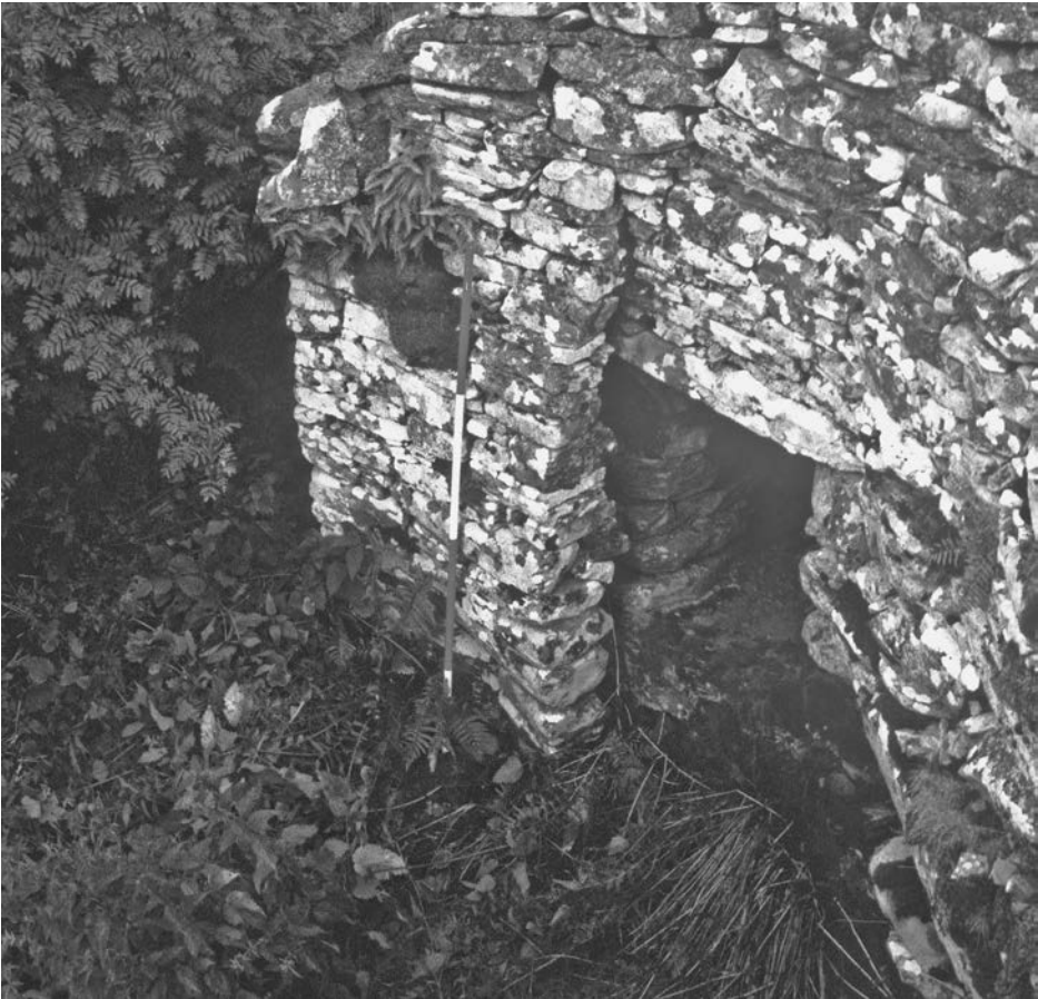
FIGURE 10.6 Post-broch secondary structures, A (above), Carn Liath, Sutherland; B (below), Ousedale, Caithness
