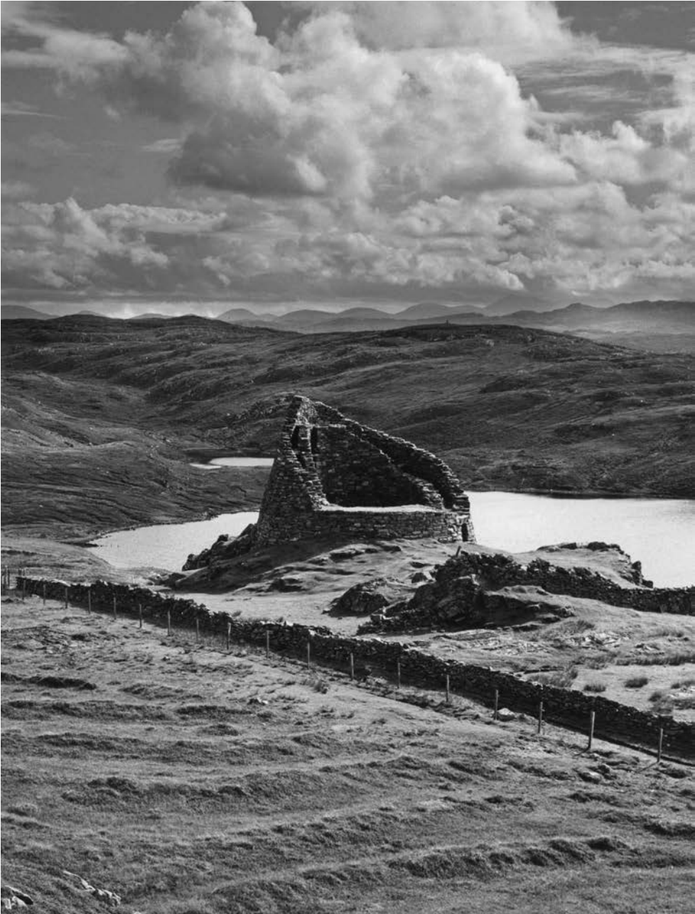
FIGURE 5.1 Carloway, Lewis, complex Atlantic round-house
