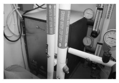
**FIGURE 2.7** Ground source water to air heat pump of ZØE lab.
