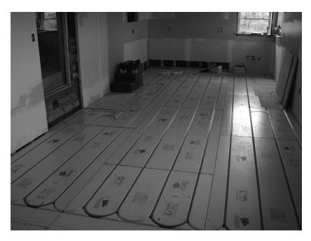
FIGURE 7.4 Warmboard radiant heat floor. (From http://www.builditsolar.com.)
