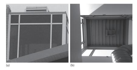
**FIGURE 2.3** The solar chimney of ZØE Lab: (a) exterior view; (b) interior view from below.
