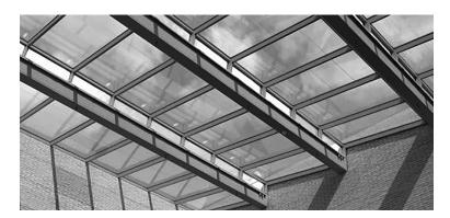
FIGURE 6.11 Semi-transparent modules. (From http://www.onyxsolar.com/photovoltaic-double-glazed-insulating-units.html.)
