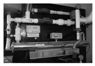
**FIGURE 2.11** The water filtration system of the ZØE Lab.
