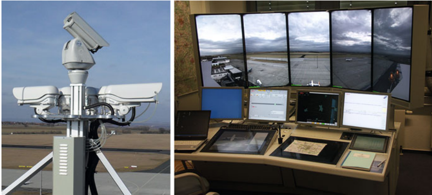
Fig. 1 Remote tower installation with 200° panorama and pan-tilt-zoom camera sensor system at the tower roof ( left photo ) and operators' workplace with 40" HD-format displays ( right ). Reprinted from (Fürstenau et al. 2013), with permission
