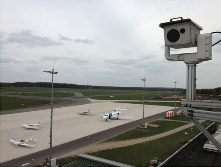
Fig. 10 FLIR thermal imager (large circular Ge-window) as part of the DLR-RTO system at Braunschweig airport, integrated in a remotely controlled housing together with visual PTZ camera
