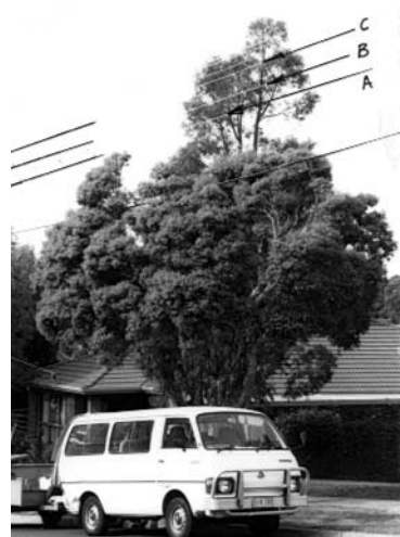
Figure 6.14 Power cables outside 72 Warburton St. A = 415 V; B = 22 kV; C = 66 kV
