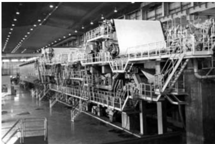
Figure 2.75 General view of a typical paper machine installation
