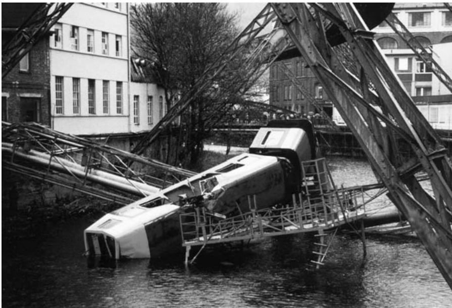
Figure 1.3 The collapse of the Wuppertal suspended railway in 1999 following incorrect installation during maintenance
