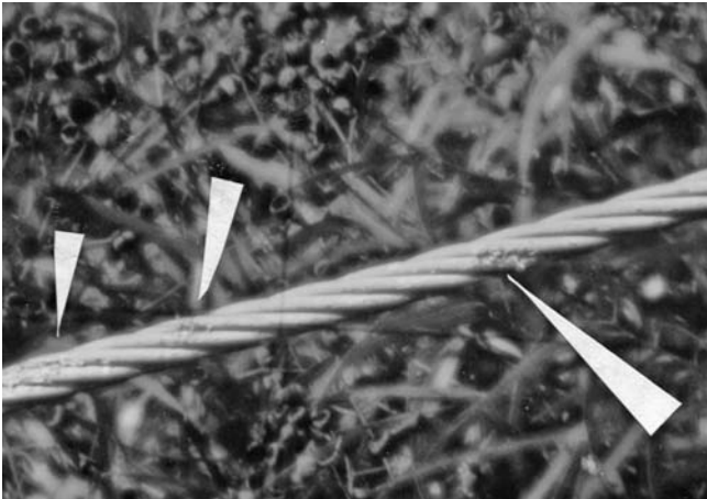
Figure 6.12 Spark-eroded section of 22 kV cable. Photo taken through theodolite telescope
