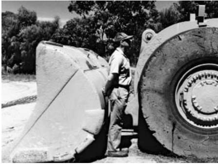
Figure 4.30 Bucket lowered and tilted forward (man approximately 1.8 m height)
