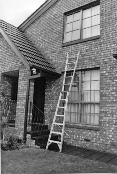
Figure 6.22 A ladder leaning against the Papgeno house. Note the steep roof above the porch (photo taken in 1997)
