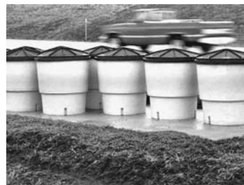
Figure 5.20 An alternative type of hollow plastic traffic barrier
