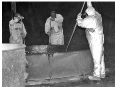
Figure 3.31 Roll-out of the FRP matrix
