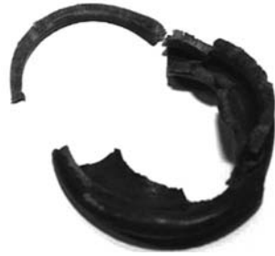
Figure 2.74 Sealing boot parts recovered from the failed joint
