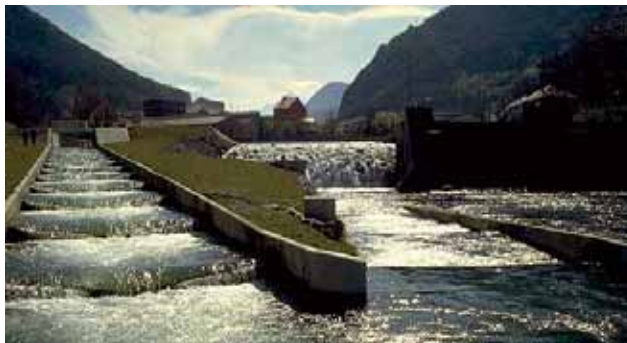
Photo 4. Pool fish pass at Sarrancolin dam (Photo Larinier)
