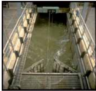
Photo 8. Holding pool and fish lift (left) and transport facility (right) (Photo Larinier)
