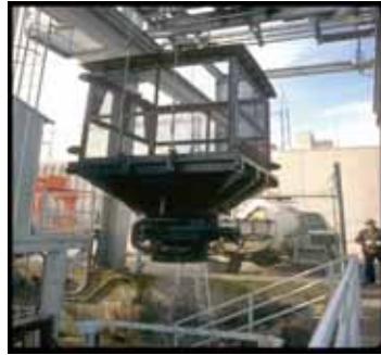
Photo 8. Holding pool and fish lift (left) and transport facility (right) (Photo Larinier)
