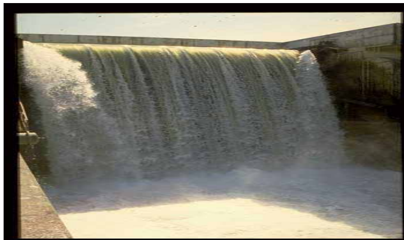
Photo 3. Spillway on the Garonne river (France)
