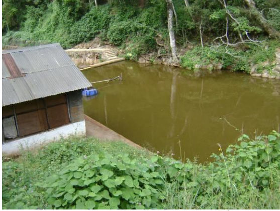
Plate 13: Bakuli 1 of Capacity 870m 3 and Silted
