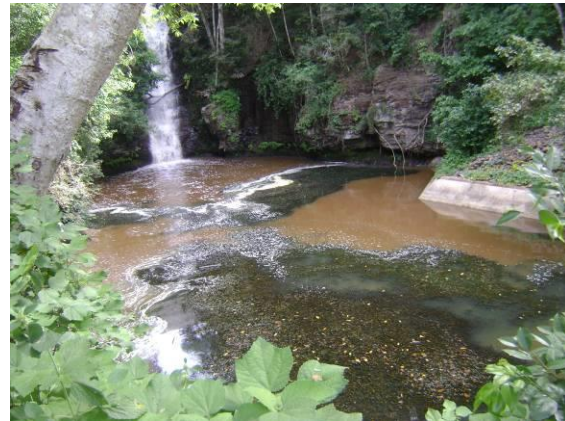
Plate 2: Silted Bakuli 2 of Capacity 570m 3
