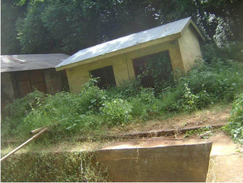
Plate 6: Abandoned Bakuli 1 pump house
