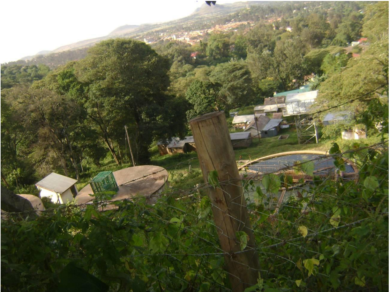
Plate 8: Existing Treatment Plant
