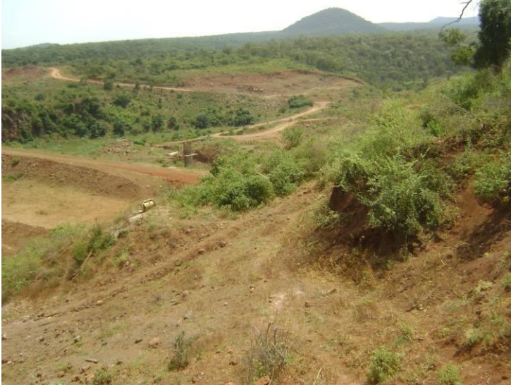
Plate 18:Badasa dam area with intake tower
