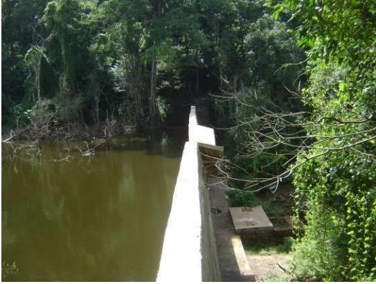
Plate 15: Rear Elevation of Bakuli 3 Dam Spillway
