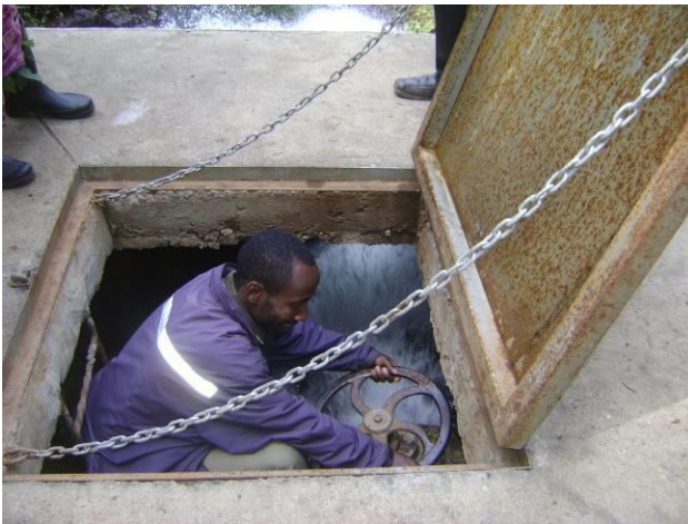
Plate 5: Bakuli 3 Dam Intake being opened
