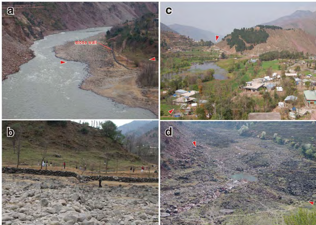
Figure 10. (a) Distant view of the surface rupture across the Jhelum River at Dhallan (location 405). Looking northeast. A scar indicated by arrows is a fault scarp formed during the 2005 earthquake. The fault scarp also crosses a man-made stone wall on the left bank. (b) Close-up view of the displaced man-made stone wall. Vertical separation is \sim 1.7 m including a broad warp on the upthrown side. (c) Distant view of Sar Pain (locations 435–442). Looking northwest. Uphill-facing warps and scarps reestablished the once-drained, dammed-up ponds, creating one of the most spectacular landscapes of the 2005 surface faulting. Given the probable presence of thick, fine-grained, dammed-up sediments, Sar Pain might serve as an excellent paleoseismic site for future studies. The inferred trace of the main rupture is indicated by arrows. (d) The tectonic bulge across the riverbed of Baghsar Katha (locations 455–459). Looking south. A small pool is formed immediately upstream of the surface rupture.
